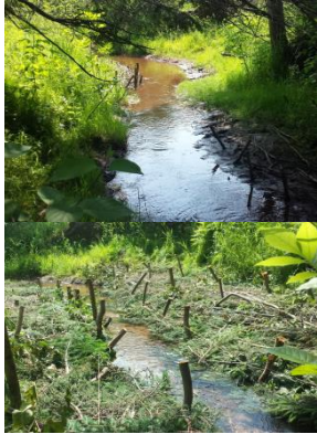
Figure 2. Before and after photos of two brushmats constructed on MacLauchlin Branch.
